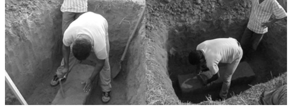
Figure 1 – Digging the hole and preparing the sample (photo: sample 1 – Cachoeira Paulista – 01/08/2002)
